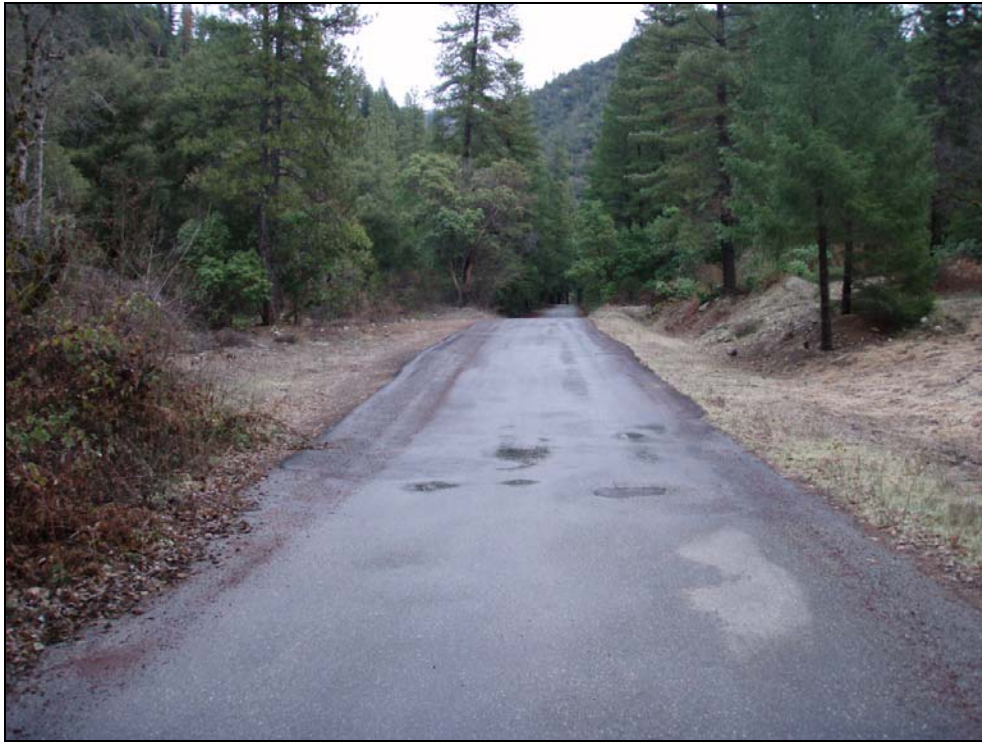
Photo 7. View east up the Cecilville Road; standing at the west channel crossing and looking towards the Hotelling Gulch stream crossing (hump in road).
