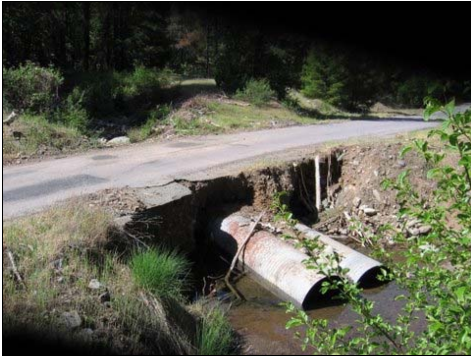
Photo 1. The Hotelling Gulch stream crossing inlet basin after significant storm damage during the winter of 2006.
