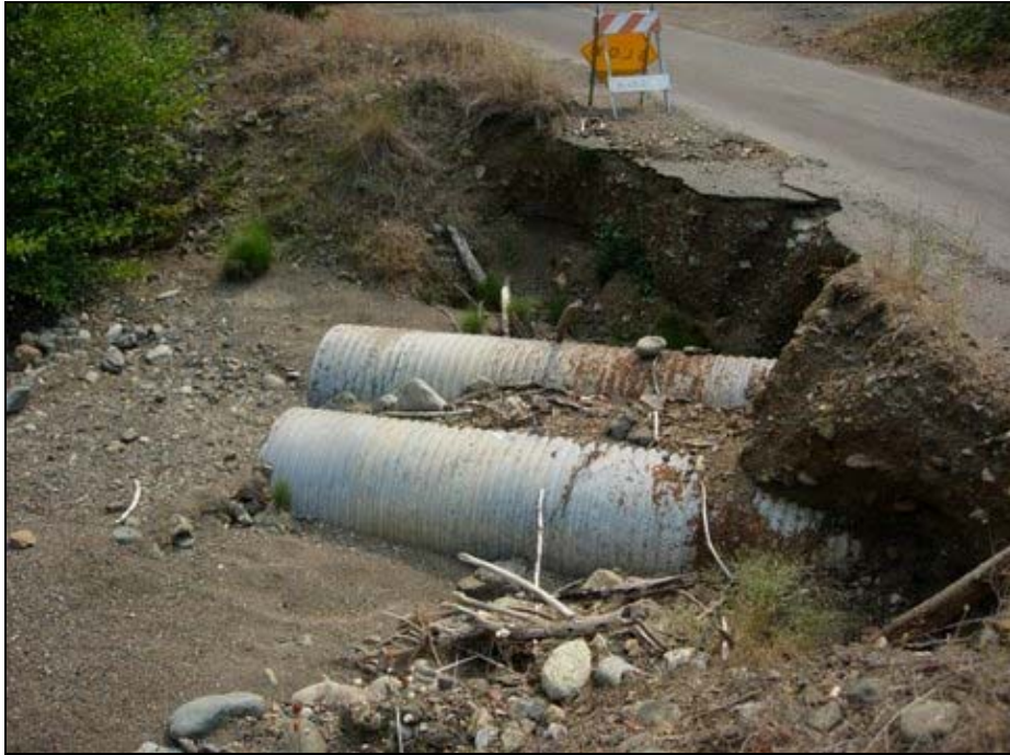
Photo 3. The Hotelling Gulch stream crossing culvert outlets after significant storm damage during the same event as Photo 1 above. Note the recent erosion of the crossing fillslope and sediment deposition filling the channel below.
