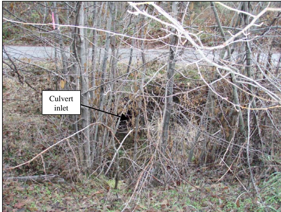
Photo 9. View of culvert inlet basin on the west channel Cecilville Road crossing. Willows constrict view.
