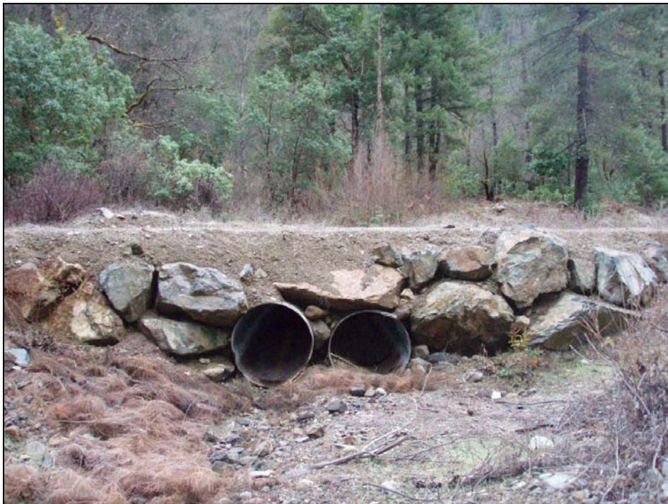
Photo 4. Current view of the culvert outlets on the existing (east channel) Cecilville Road crossing.
