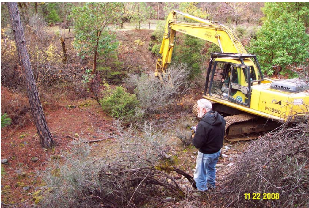
Photo 12. Getting ready to start a new excavation pit along the west alignment above the Cecilville Road.
