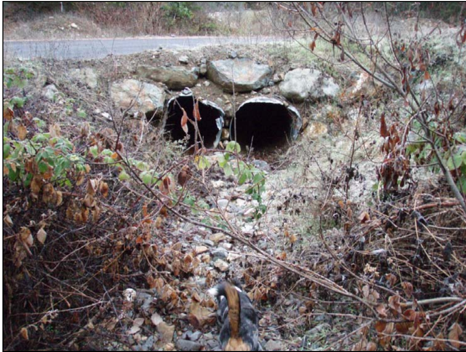
Photo 2. Current view of the inlet basin on the existing (east channel) Cecilville Road crossing.
