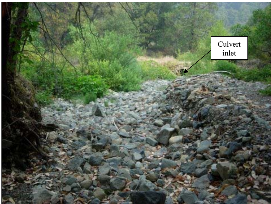
Photo 6. The active stream channel looking downstream at the Hotelling Gulch stream crossing, approaching the culvert inlet basin. Note the recent terrace deposits to the right, likely caused by culvert plugging and backwatering of the stream crossing.
